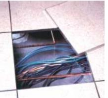
Placed in the subfloor of a computer room, the TraceTek system protects your computer equipment by detecting a leak early – and even locating its source.
